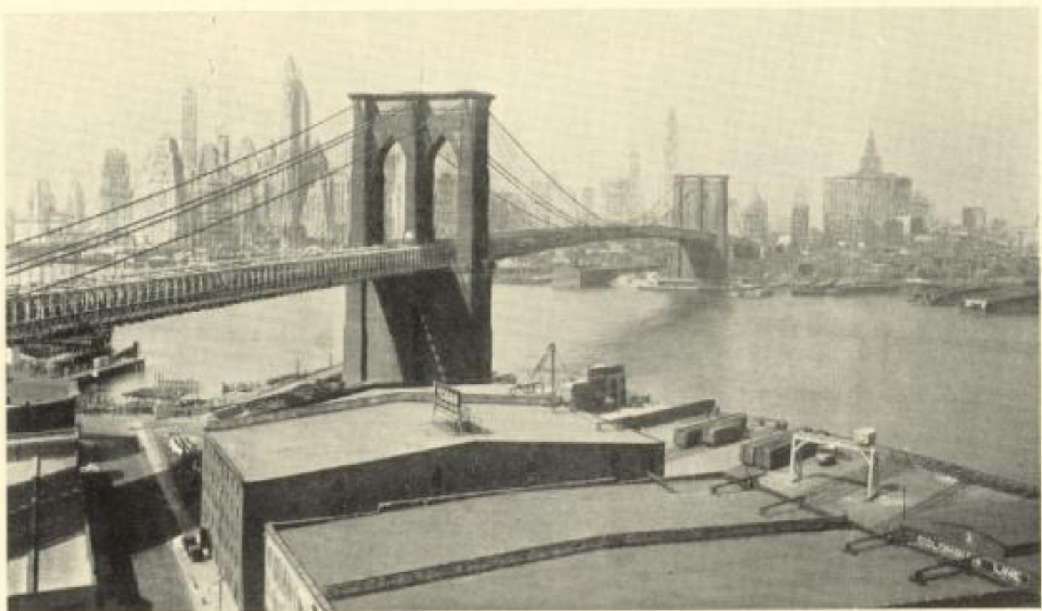
Brooklyn Bridge looking toward Manhattan—1933.
