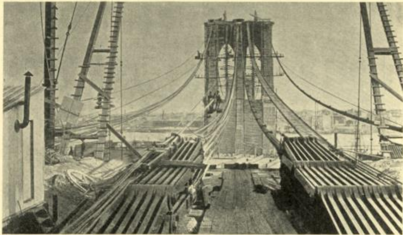
Brooklyn Bridge. Wire cables under construction. Last cable wire was run October 5, 1878.
